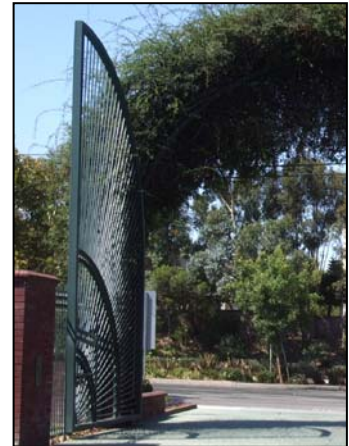
Entrance detail, El Toro Memorial Park
